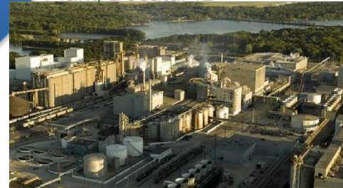
Construction complete – Operational Jan 1 2017
